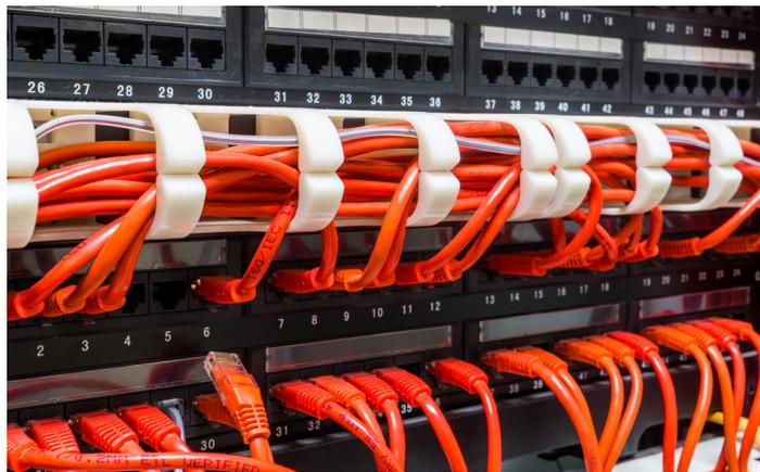
**Figure 3:** Data centers – with their enormous amount of cabling – are particularly susceptible to catastrophic fires. The adoption of LSZH cabling can make a world of difference in these environments. (Source: Adobe Stock)
